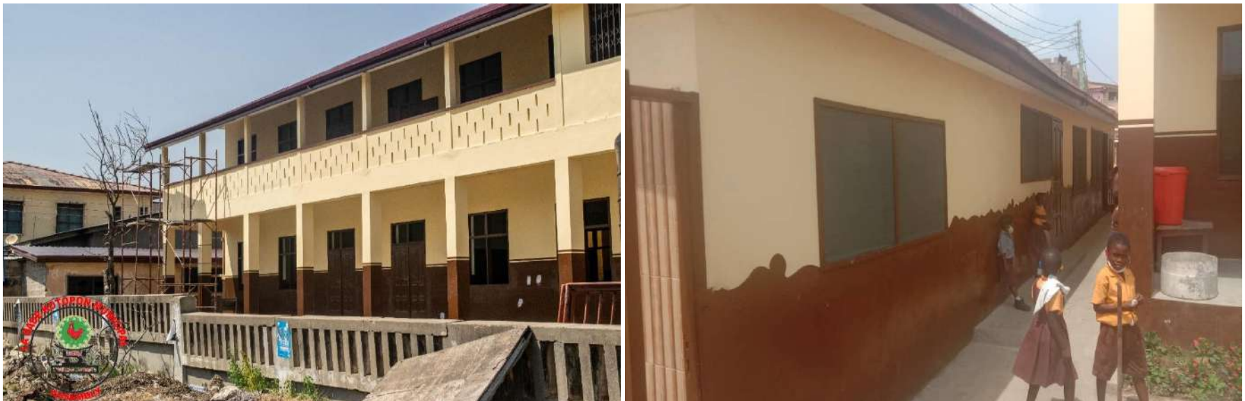
Figure 1.6 Rehabilitated 2-Storey 6-Unit and 4-Unit Classroom Block at South La
