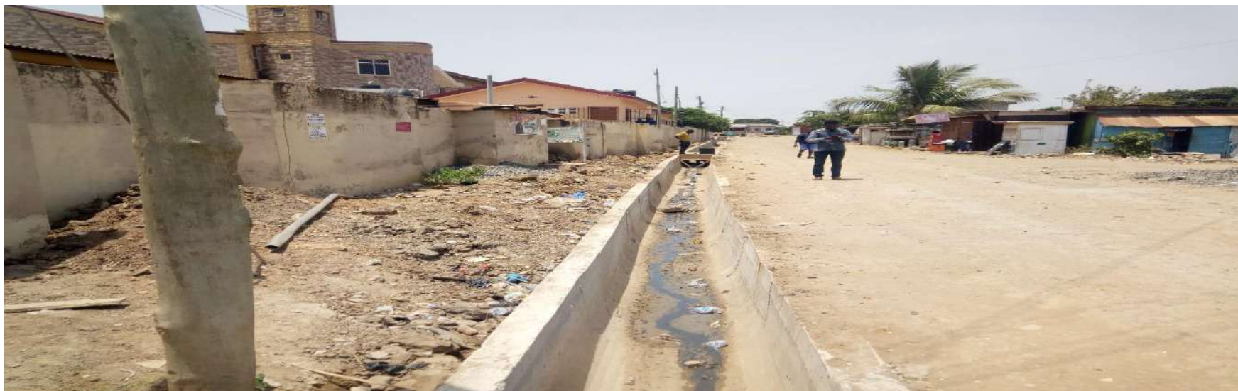
Figure 1.7 COMPLETED 0.9M U-DRAIN FROM NAVITY TO KENAM FACTORY
