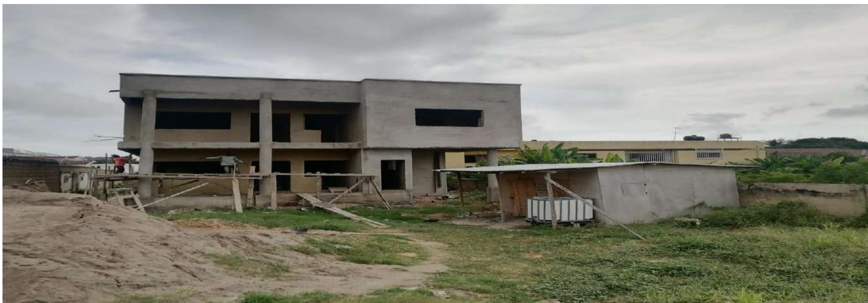
Figure 1.8 COMPLETION OF 2-STOREY 4-BEDROOM BUNGALOW FOR MCE AT LABONE
