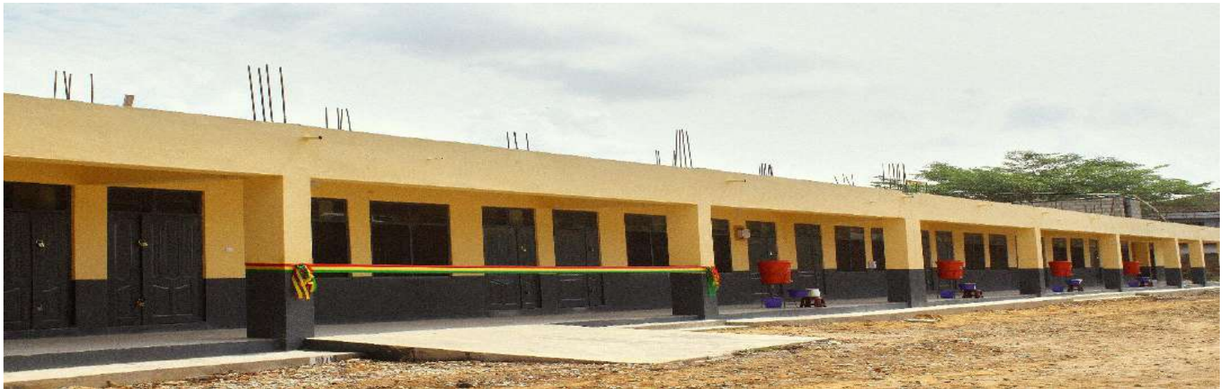
Figure 1.5 COMPLETED 1NO. 6-UNIT CLASSROOM BLOCK WITH ANCILLARY FACILITIES AT ASSOCIATION SCH. LABONE
