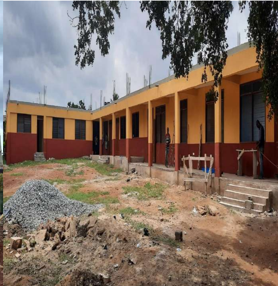
COMPLETION OF 1NO. 6-UNIT CLASSROOM BLOCK WITH ANCILLARY FACILITIES
