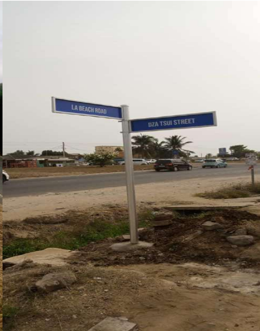
INSTALLATION OF STREET NAMES
