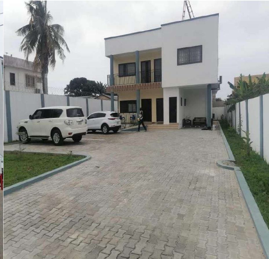
COMPLETED 2-STOREY 4-BEDROOM BUNGALOW FOR MCE
