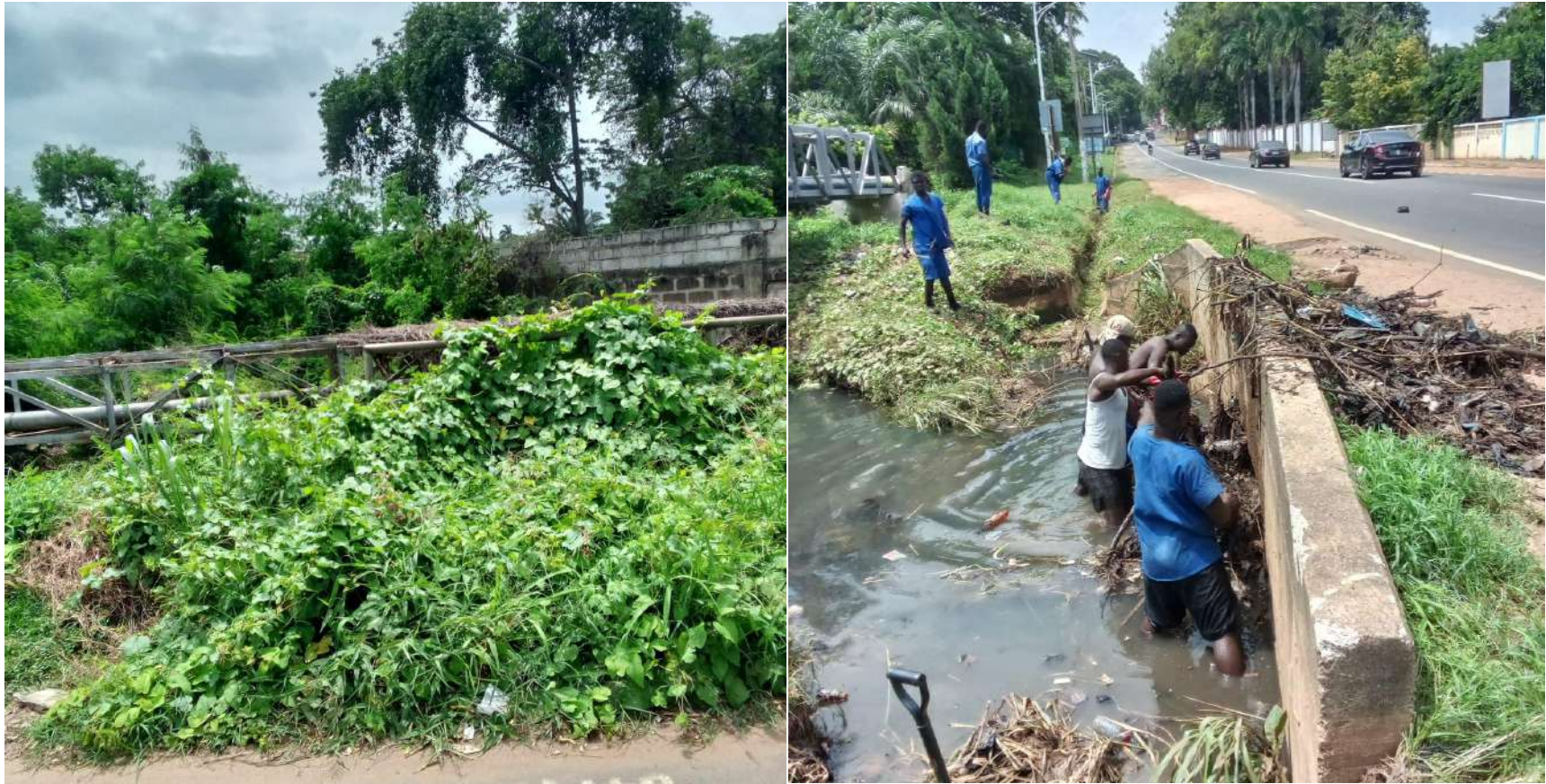
DESILTING OF EARTH & CONCRETE DRAINS (BEFORE & AFTER)
