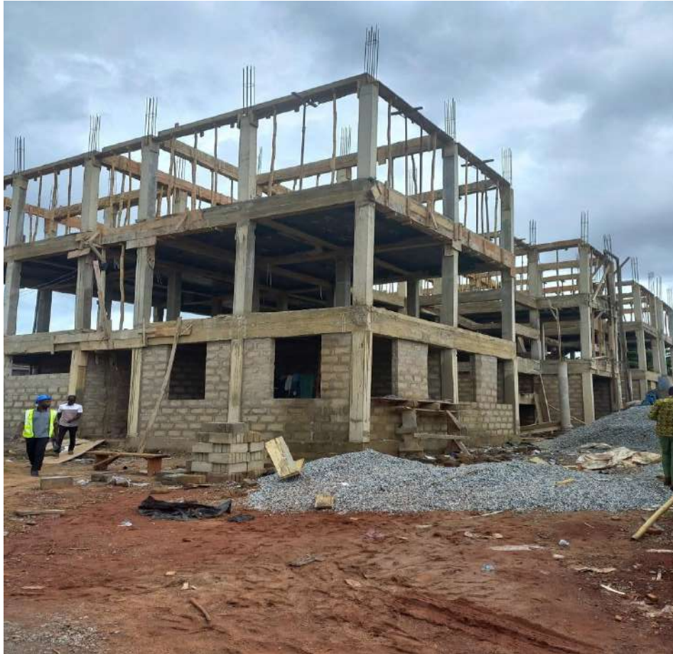
COMPLETION OF 1NO 3-STOREY 18-UNIT CLASSROOM BLOCK WITH ANC. FACILITIES
